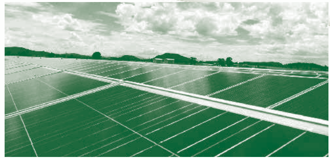
PV 08 Location Phanom Thuan District, Kanchanaburi Selling Capacity 8 MW COD 6 Jun 2014
