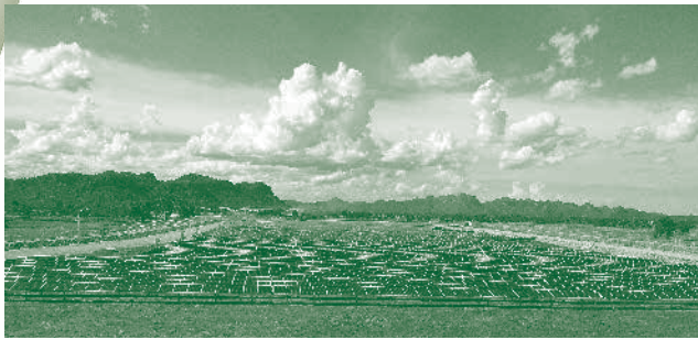
PV 07 Location Tha Muang District, Kanchanaburi Selling Capacity 8 MW COD 20 Mar 2014
