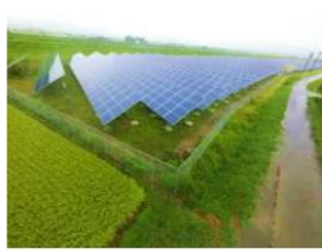
Shima (1.25 MW) COD MAR 2016
