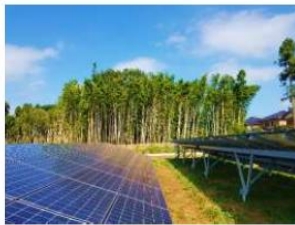
Jyoso (1.25 MW) COD MAY 2018
