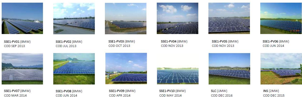
Figure 1: TSE solar farm in Thailand
