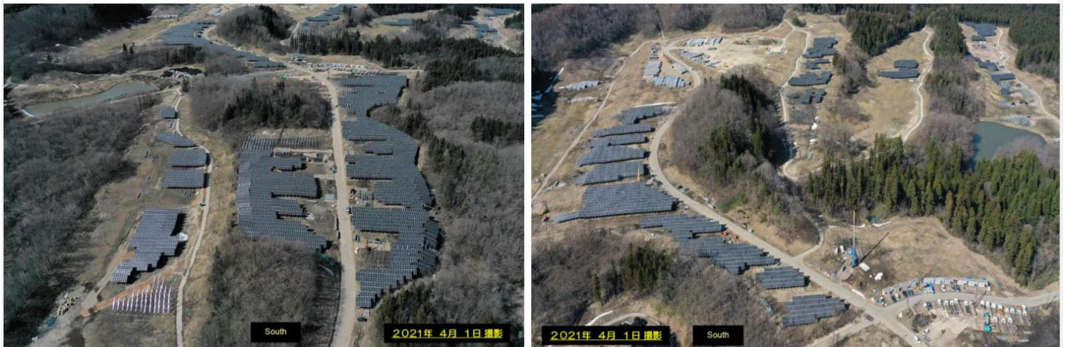
Fig 3: Progress of Onikoube Project: 30% completion at the end of 1Q21 and is expected approximately 70% at the end of 2021E
