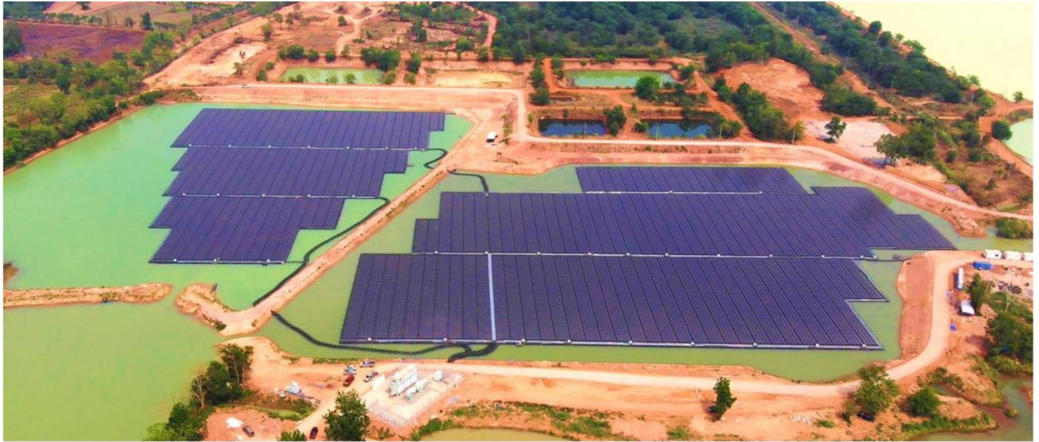
Fig 2: Floating Solar Project is started on schedule
