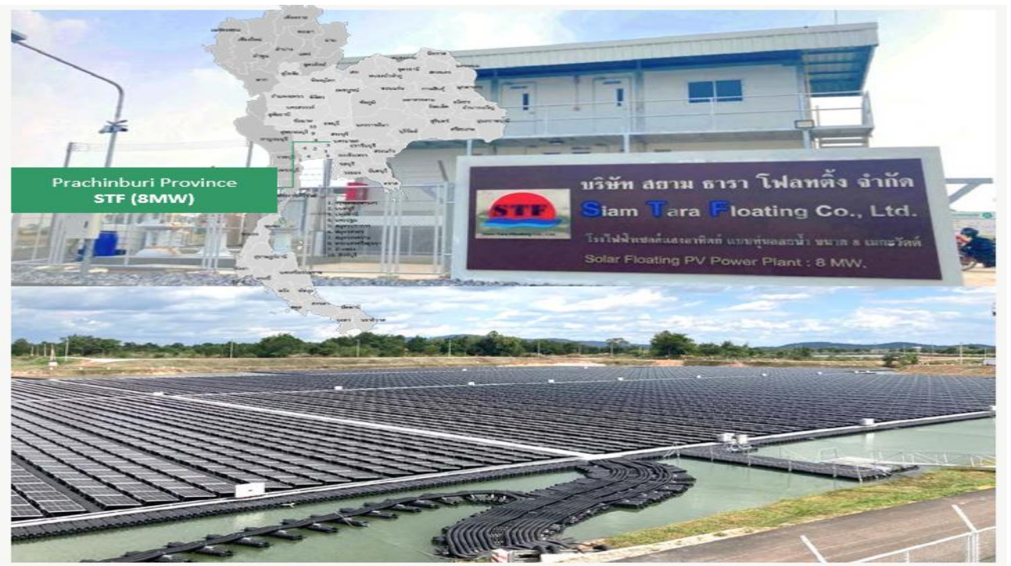
Fig 3: Floating Solar Project “Siam Tara Floating” with 100% Offtake from Hitachi in Kabinburi Industrial Estate
