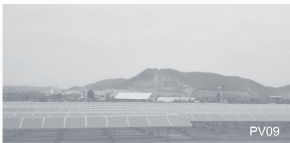
Location U-Thong District, Suphanburi Selling Capacity 8 MW COD 4 Apr 2014
