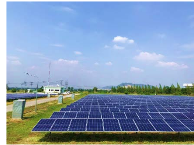
SSE1-PV09 (8MW) COD APR 2014
