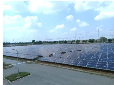
SSE1-PV02 (8MW) COD JUL 2013
