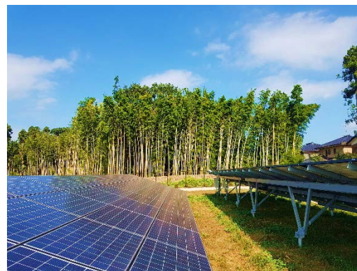
Jyoso (1.25 MW) COD MAY 2018
