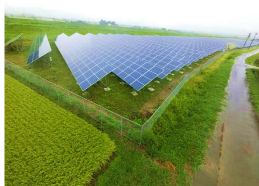
Shima (1.25 MW) COD MAR 2016
