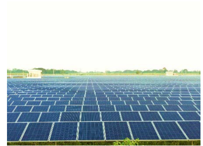
SSE1-PV10 (8MW) COD MAY 2014
