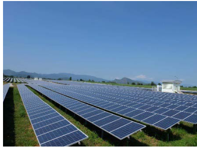
SSE1-PV01 (8MW) COD SEP 2013
