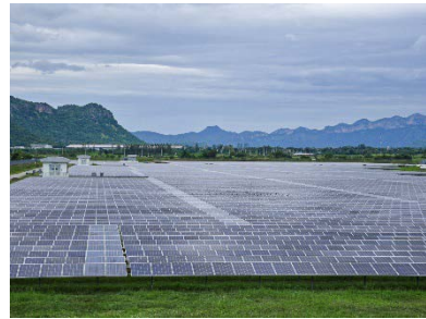
SSE1-PV07 (8MW) COD MAR 2014
