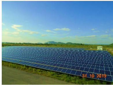
SSE1-PV06 (8MW) COD JUN 2014
