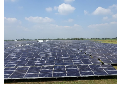
SSE1-PV05 (8MW) COD NOV 2013
