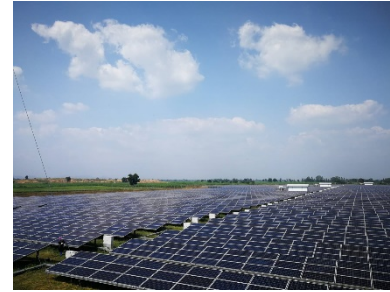
SSE1-PV04 (8MW) COD NOV 2013
