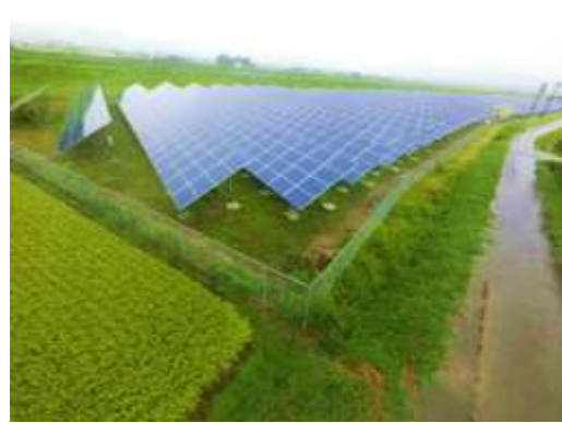
Shima (1.25 MW) COD MAR 2016
