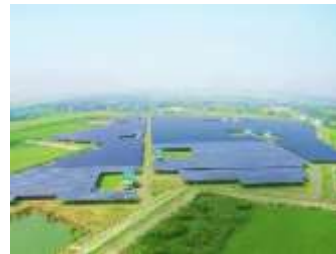
SSP (8MW) COD MAR 2013
