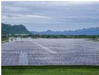
SSE1-PV07 (8MW) COD MAR 2014
