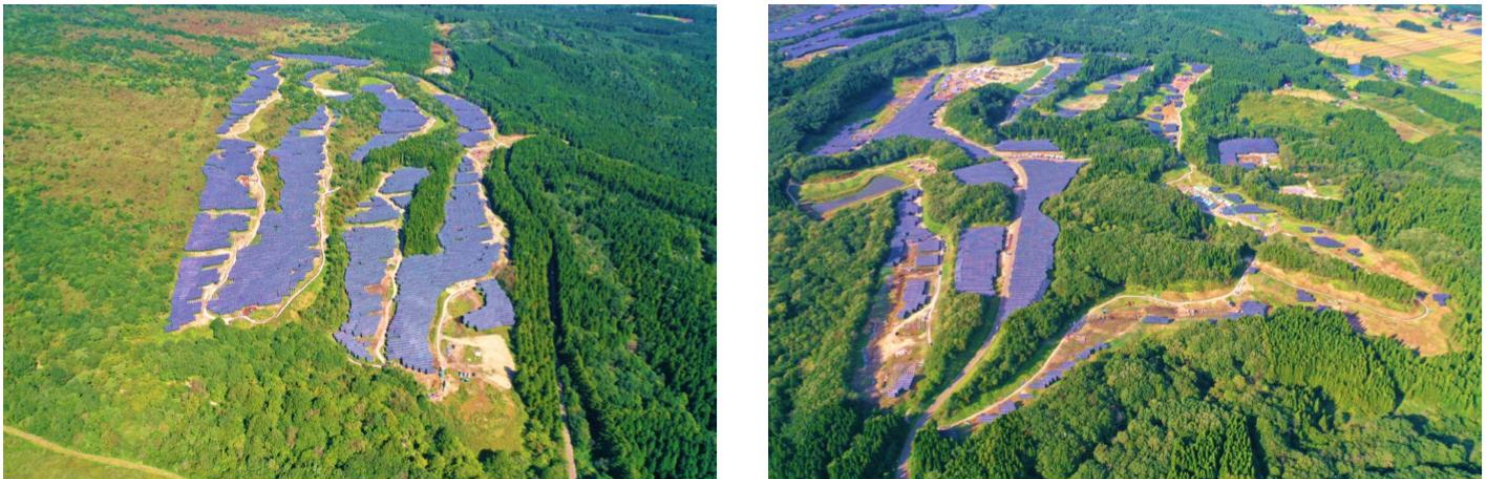
Fig 3: Onikoube Project: Remains under schedule to COD in 1Q23E
