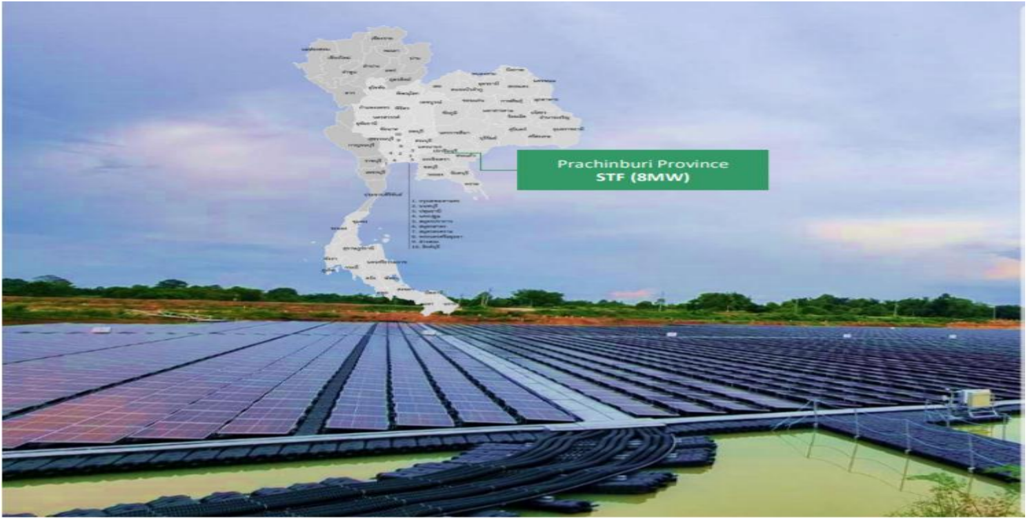
Fig 2: Floating Solar Project “Siam Tara Floating” with 100% Offtake from Hitachi
