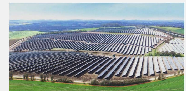
Ref. photo of "Onikoube" project
