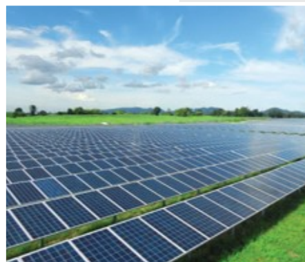
Solar PV Farm
