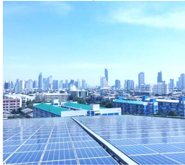
Solar PV Rooftops
