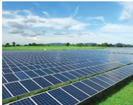
Solar PV Farm
